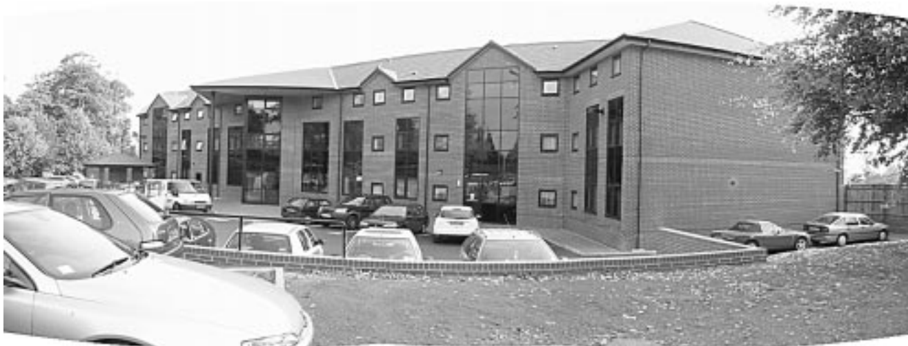
StowHealth is the first building in Suffolk with health and social care provision under one roof. Opened in September 2003, it is spacious and the staff are friendly and efficient. A changing exhibition of paintings (which can be purchased) by local artists is displayed in its public areas. For more information see www.stowhealth.com
